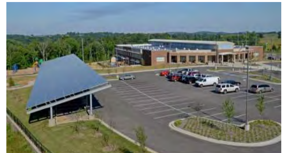
Image Credits: CMTA Engineers
