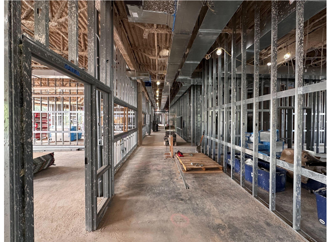
Wall Framing and Rough-ins in a Typical Corridor
