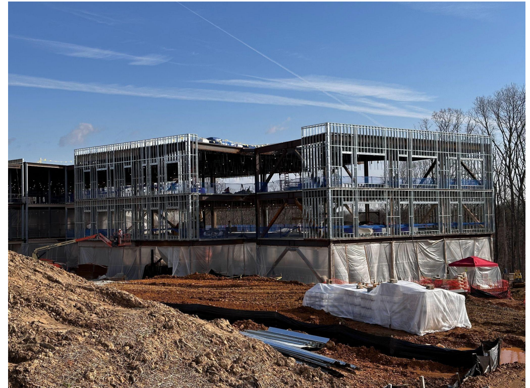
Southwest Corner of the Classroom Wing
