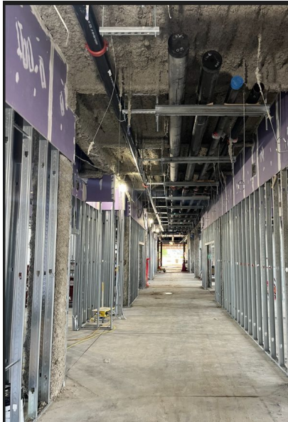
Spray on Fireproofing Interior Framing MEP Overhead Rough In
