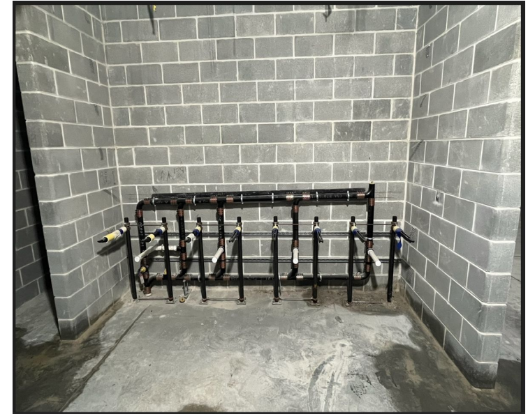
Locker Room Bathroom Plumbing
