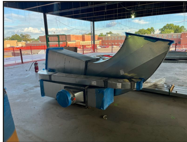
Mechanical, Electrical, Plumbing and Fire Suppression Fitout
