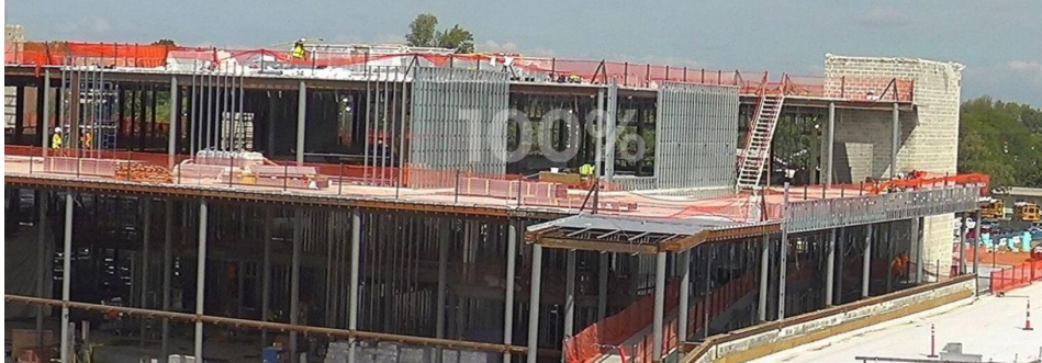
Exterior Framing South
