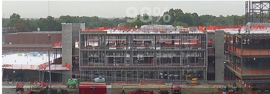
Exterior Framing North
